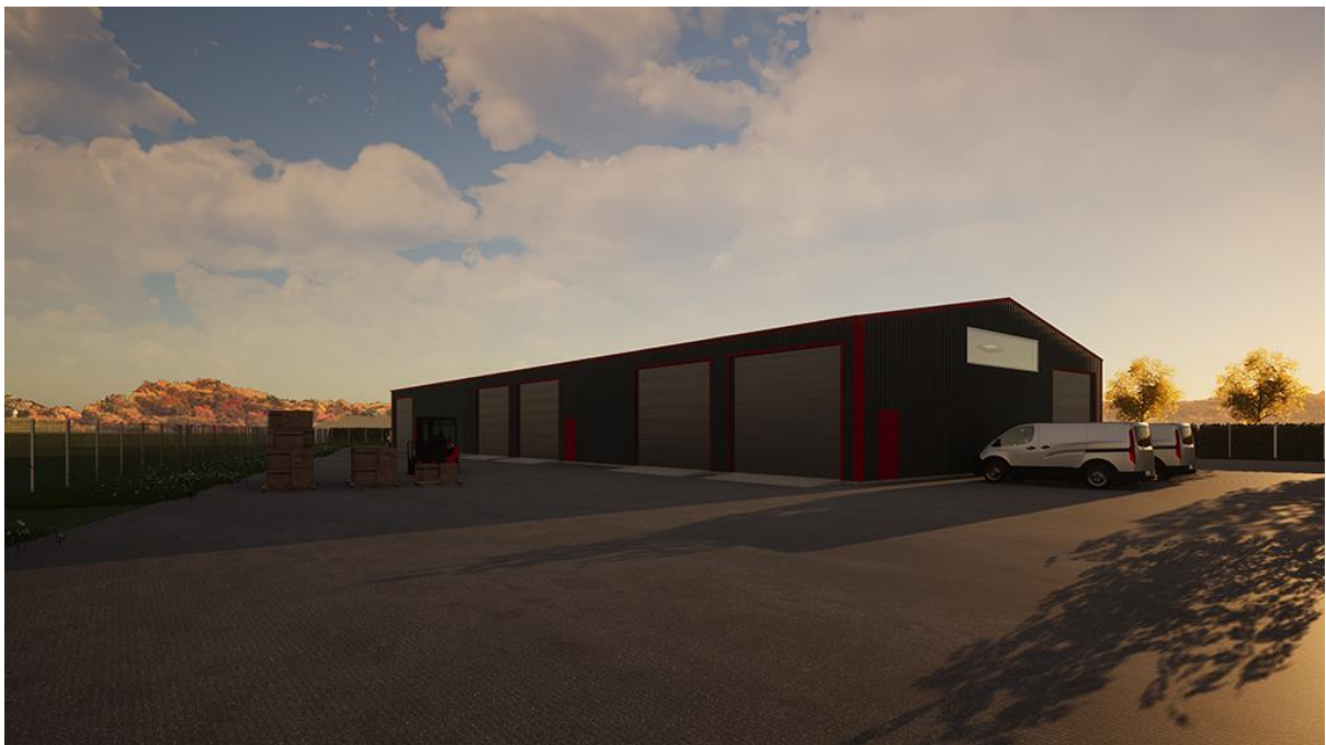
View from north west of site looking south east
