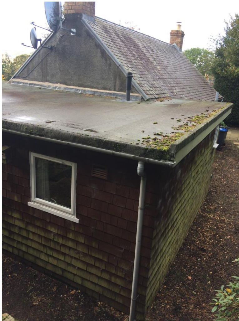
Flat Roof to Original Extension
